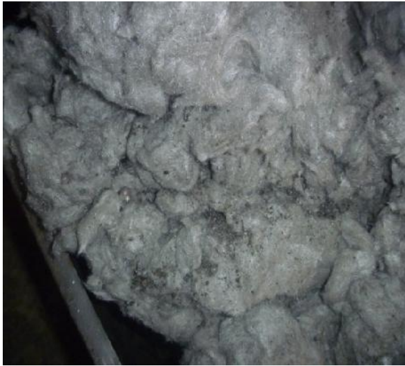
Fig. 3.2. Dumping of mineral wool inside the hollow casing
