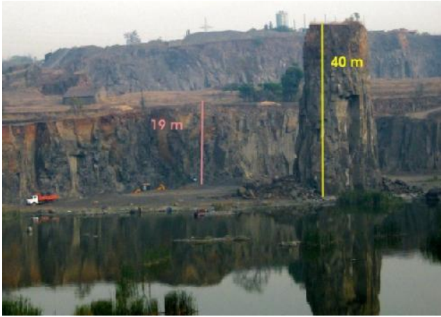
Fig. 2. Massive depth quarries with accumulated water at Top
