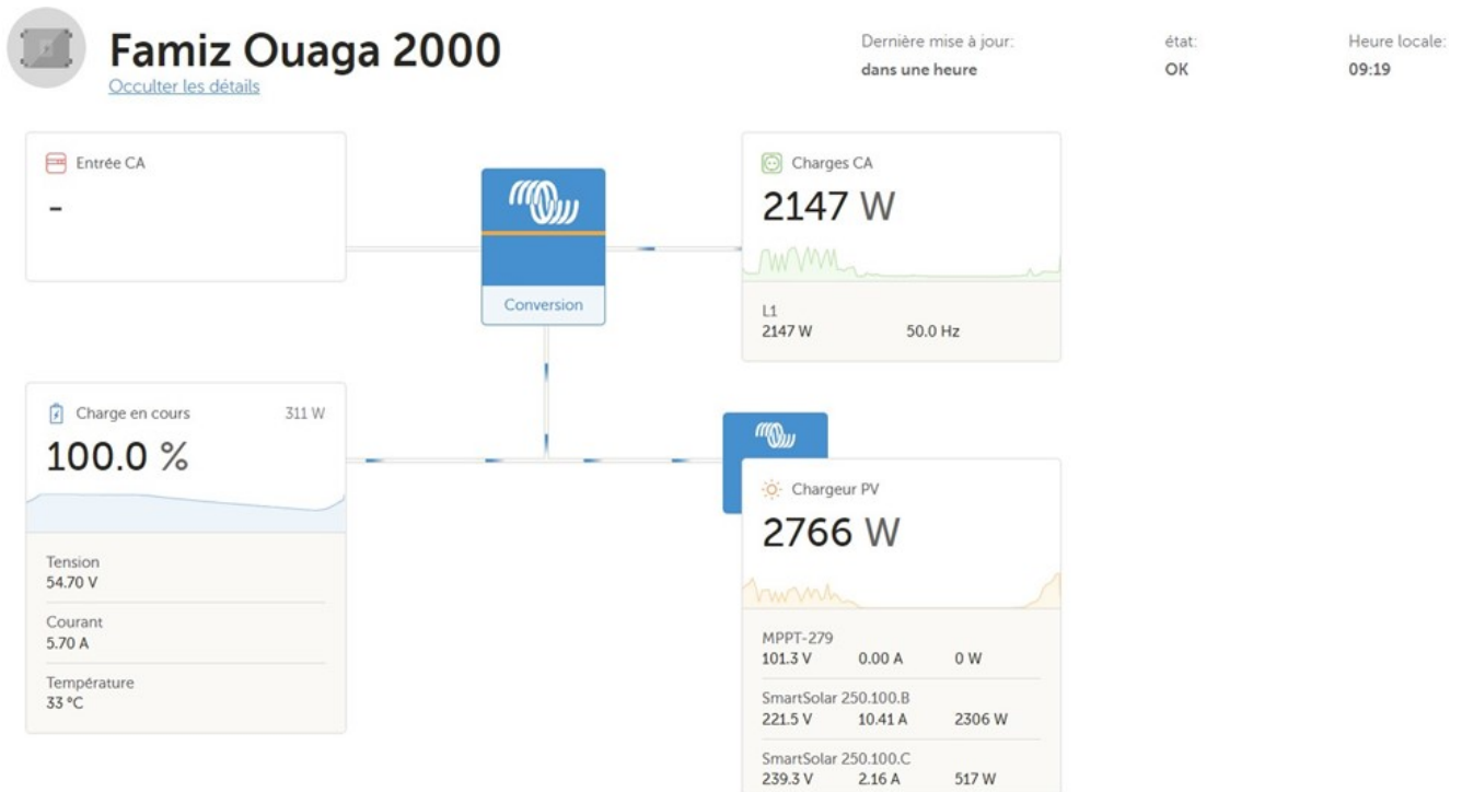
Figure 3. Installation monitoring window on 25 August 2024 on 09: 19 Am
