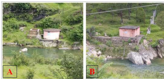
Plate 2. Typical example of lift irrigation in the Upper Kosi watershed: A- Pumping House at village Pakhura and B- Pumping House at village Kaleth
