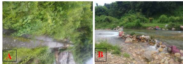
Plate 1. Typical examples of a canal in the Upper Kosi watershed at the Falta village: A-Canal and B- check dam 'band'
