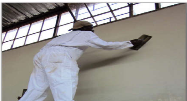
Fig. 5. Finishing of last layer
