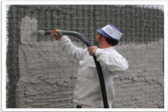
Fig. 4. Shotcrete by machine
