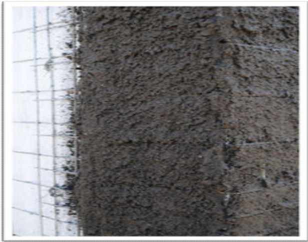
Fig. 3. First layer of plastering
