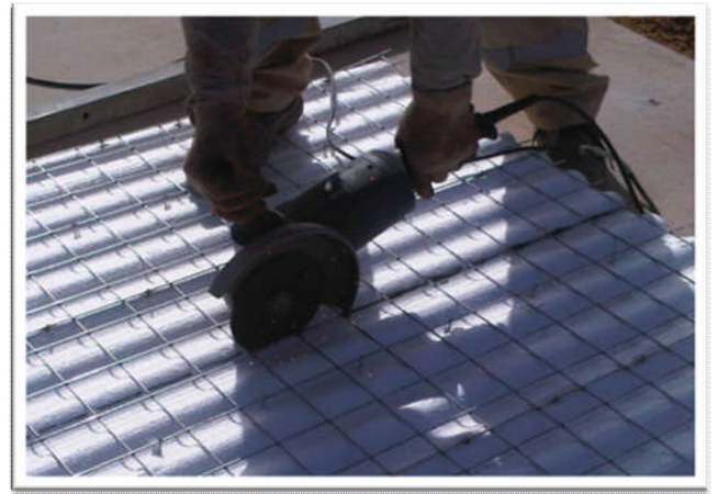
Fig. 6. Cutting of panels
