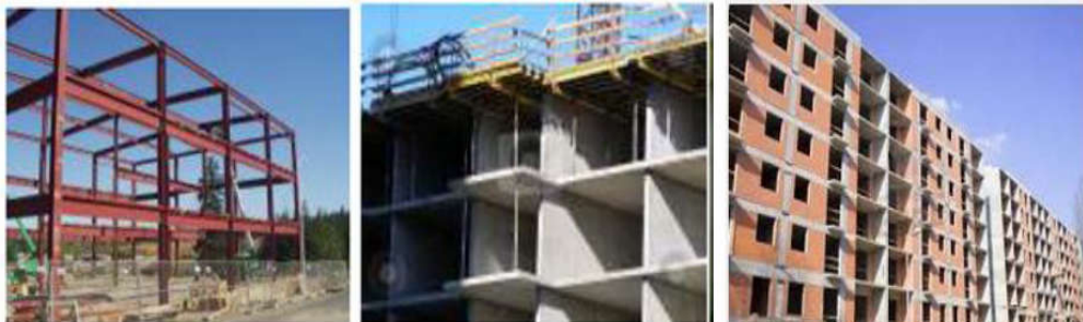
Fig.2. Moment resisting frame of shear wall and infilled frame structure
