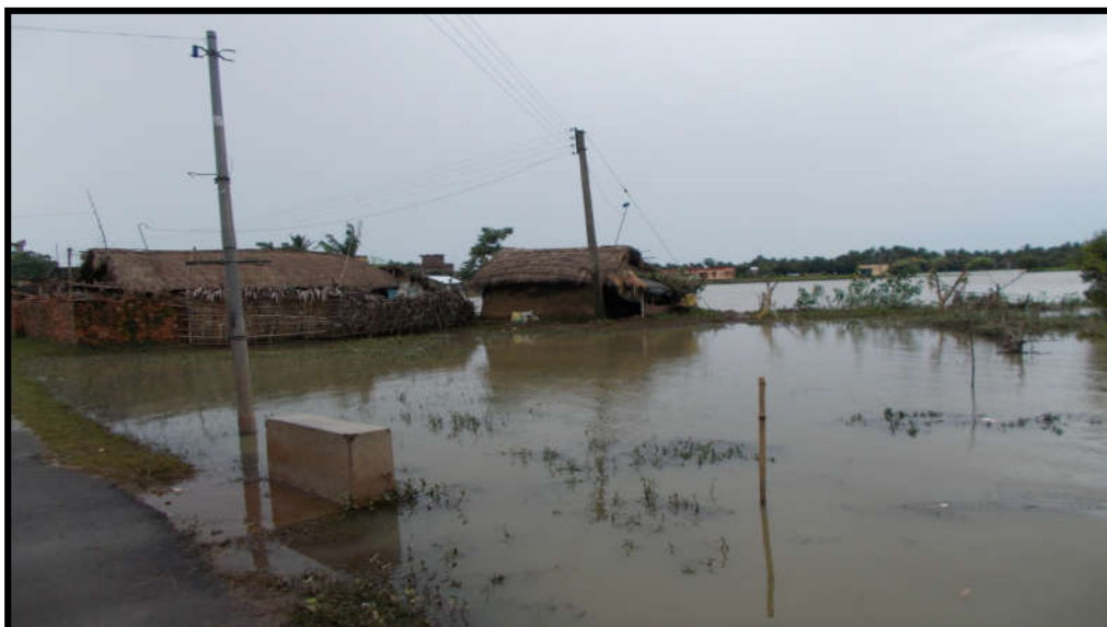
Plate 4. In a portion of Kandi block on flood's time (2015)
