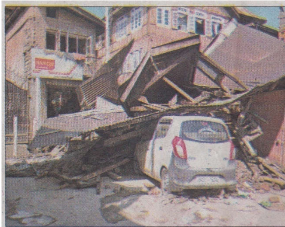
A view of a collapsed shed in Chatabal area of the old city.
