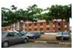
Figure 1. School of Earth and Mineral Sciences, FUT, Akure. Use of Brick facing as Wall Finishing
