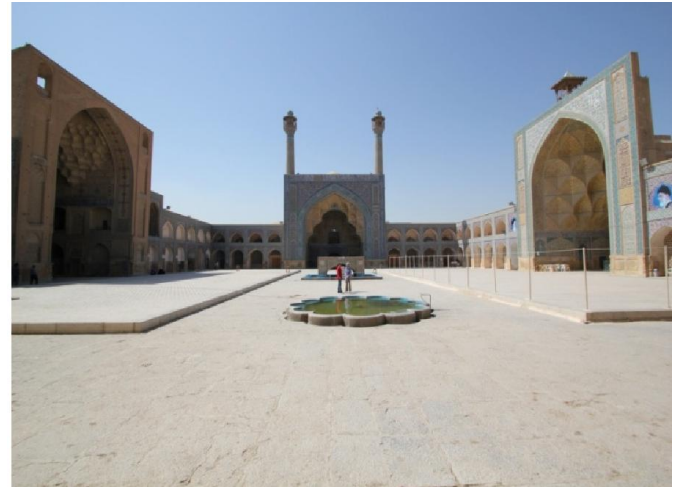
Figure 12. The Four Iwans of Mosque Isfahan, Isfahan, Iran. Retrieved 25/9/2014 from http://farflungistan.com
