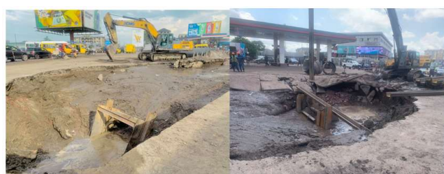
Figure 2. Landslides during the installation of DN 1400 FD pipes
