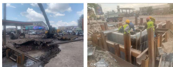
Figure 4. Sheet pile protection operations during construction work
