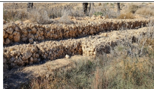
Figure 6. Stone retaining dams
