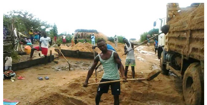
Picture 3. Loading of a truck by men, Madindé, 2022
