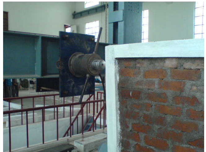
Fig: 8. loading arrangement set up (infilled frames)
