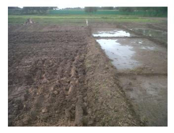
Figure 1. Expansive soils hydration by means of the "presaturation" method
