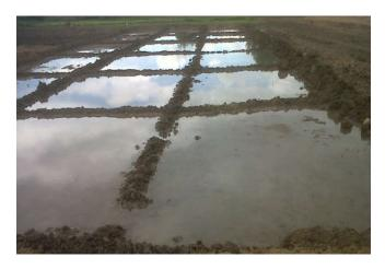
Figure 3. Expansive soil ponding by means of the "presaturation" method
