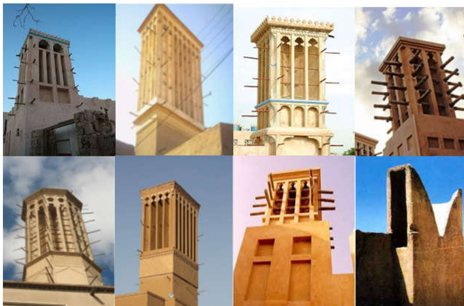
Figure 1. Wind-catcher in traditional architecture with different number of openings
